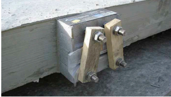
Figure 8 – Close up of cast in thermal breaks.
