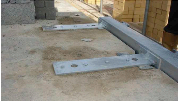
Figure 6 – Section through RC slab with L shape bracket fixed through the floor.
